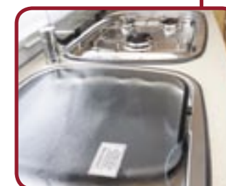
Fixed drainer, sink and hob top chopping-board-grade covers
